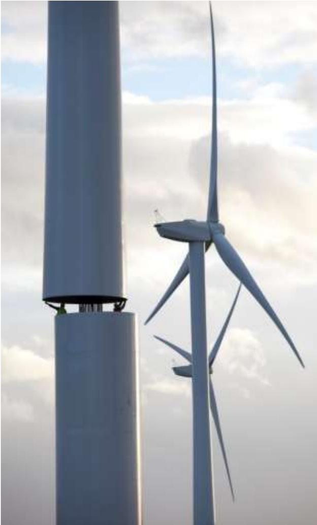
For standard 'flange-jointed' tower design, we possess full TUV Nord approval for the manufacture and supply of EN 14399-4 products in hot-dip galvanized finish in accordance with ISO 10684.
